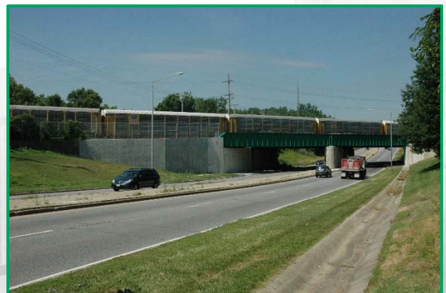
New rail bridge over 127 th Street
