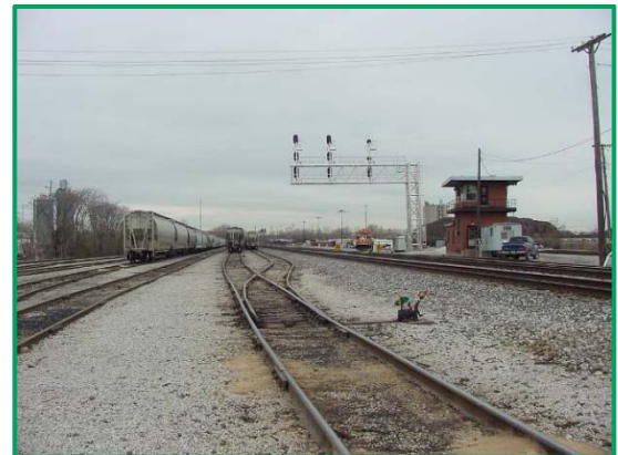
New Signal Bridge along the IHB
