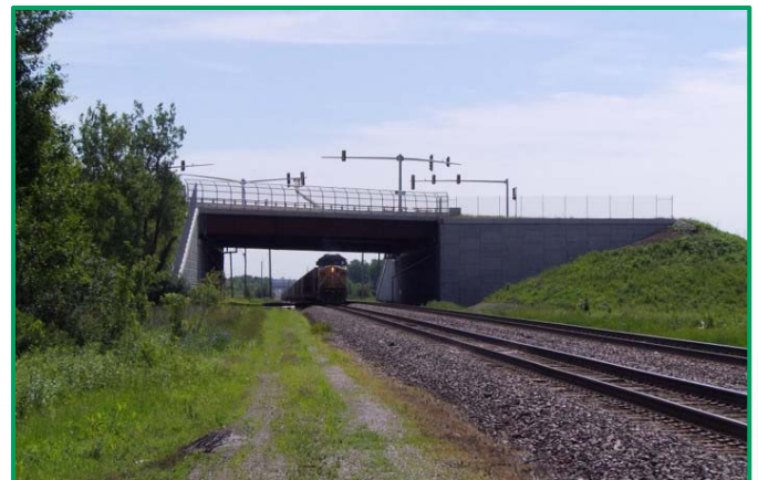
View from the west of new overpass
