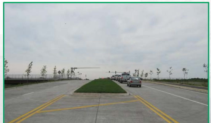
View from the north of new intersection
