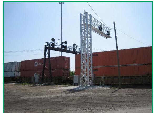
New Signal Bridge near Corwith Yard
